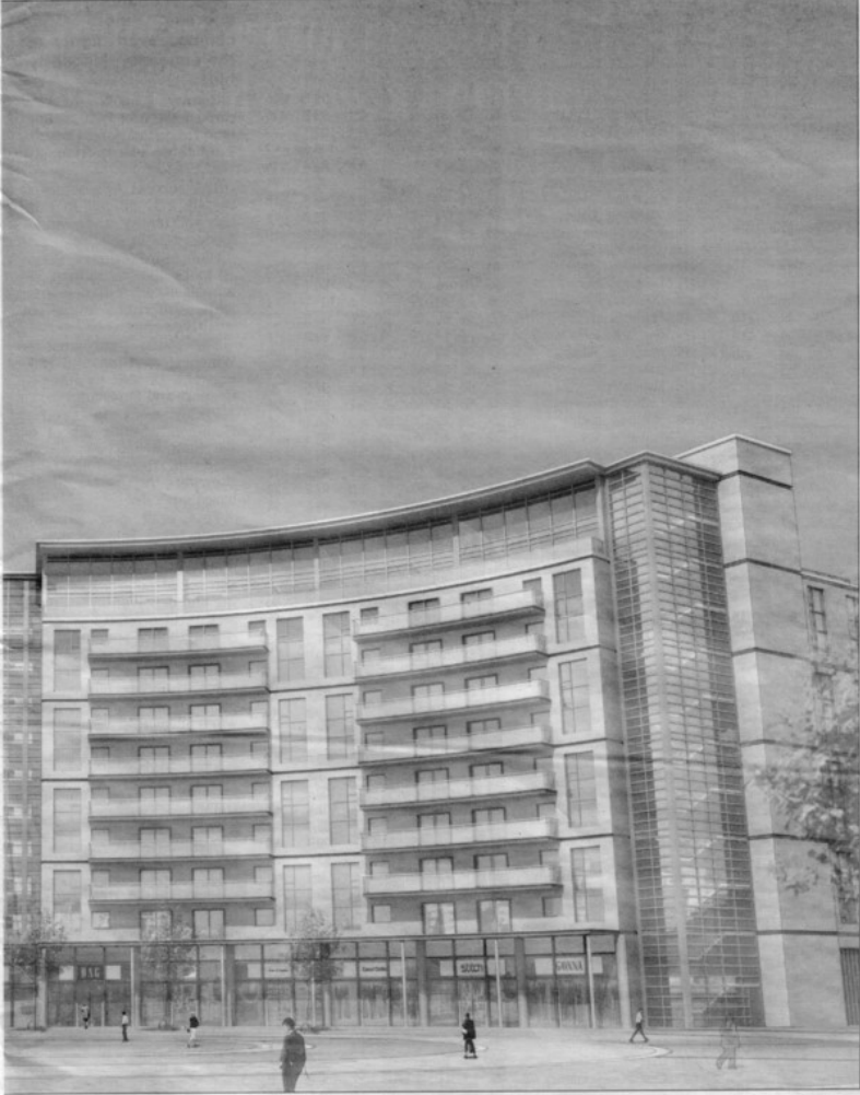
Impression, with the proposed East Side Plaza in the foreground and 12-storey crescent block, right
